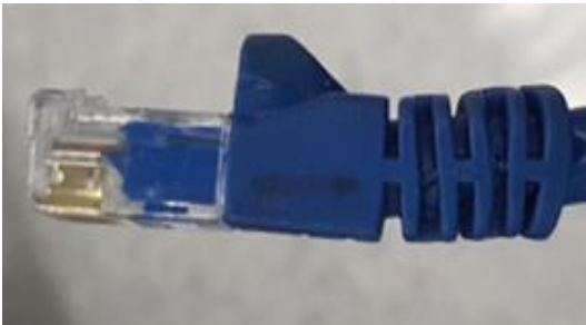
Ethernet Connector Lock – Not good Condition
