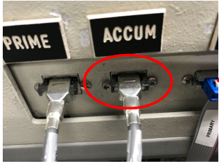
ACCUM Connector Intermittent
