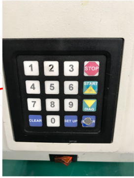
Keypad Not In Good Condition
